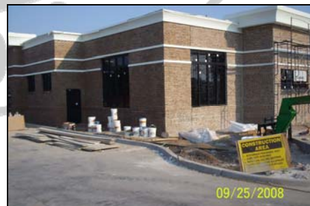
New Zaxby’s Prototype in The Colony, TX during construction
